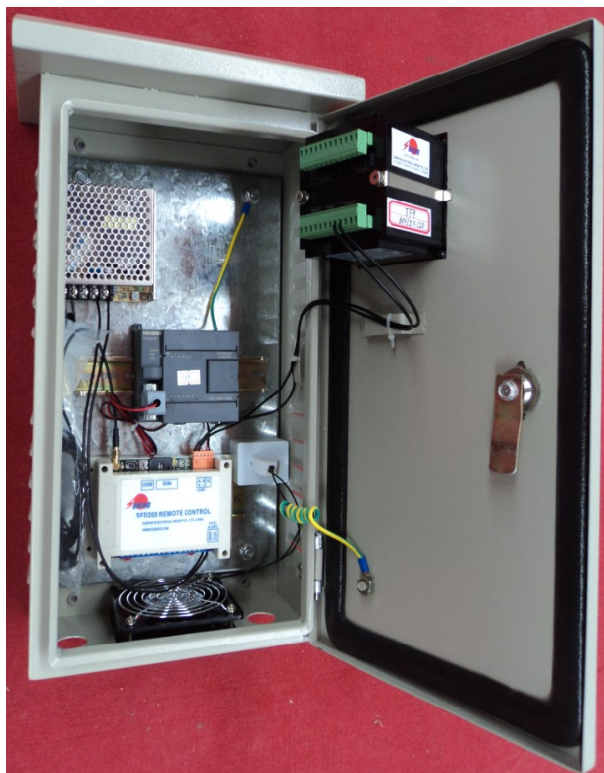
From TF1 to TF26 except TF2 and TF6 (Substation A)
